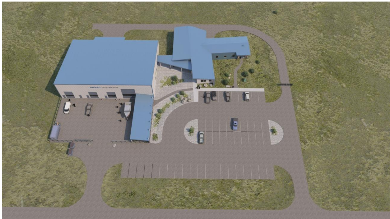
Figure 2: A bird's eye view of the completed SAVEC campus on a hypothetical site.
